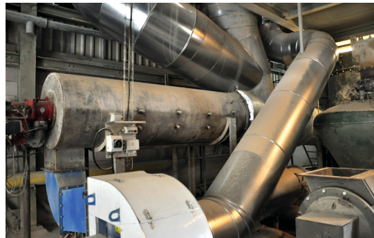
4 Hot gas generator from Gebr. Pfeiffer with new dilution air fan after the modifications of Steps 1 and 2
